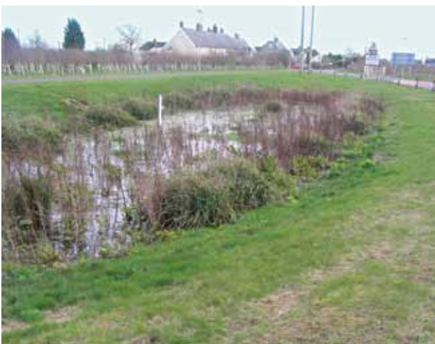
Pond drainage system alongside a road in Oxfordshire (Tony Gent)
