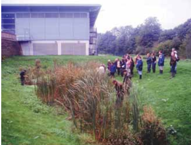
The SUDS system at Hopwood Park motorway service station includes a series of small ponds, some of which have been colonised by amphibians including the great crested newt (ARC)
