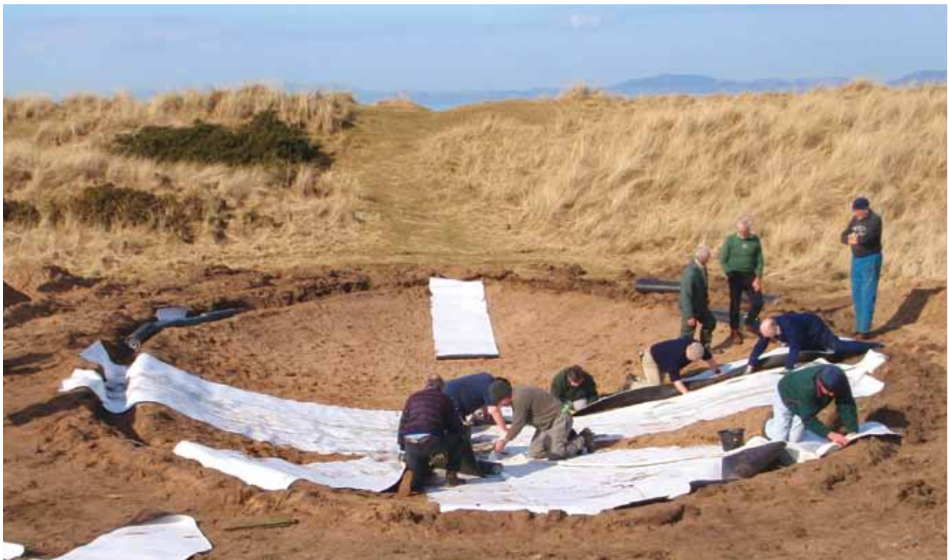
Natterjack scrape being lined with prehydrated bentonite (RAWMAT® HDB) at Mawbray Banks (Bill Shaw)
