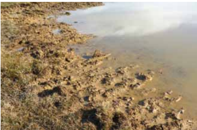
A toothed bucket on a mechanical digger leaves an uneven finish which increases microhabitat diversity in non-lined ponds (David Orchard)
